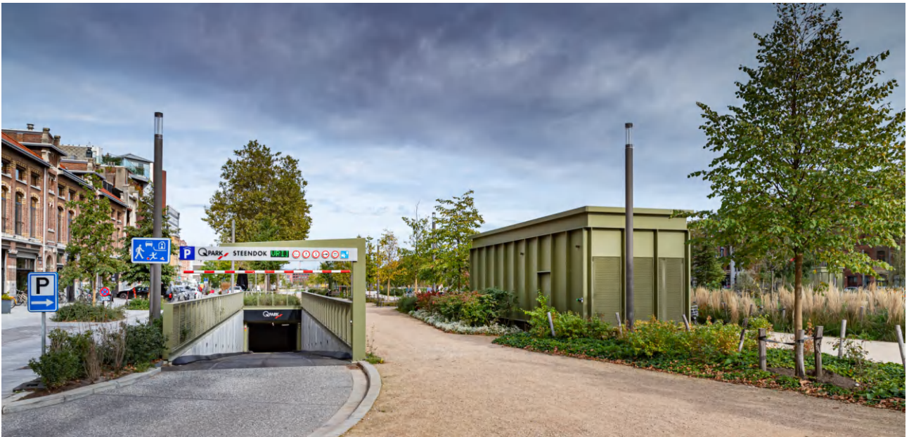
People above ground - cars and bicycles under ground
