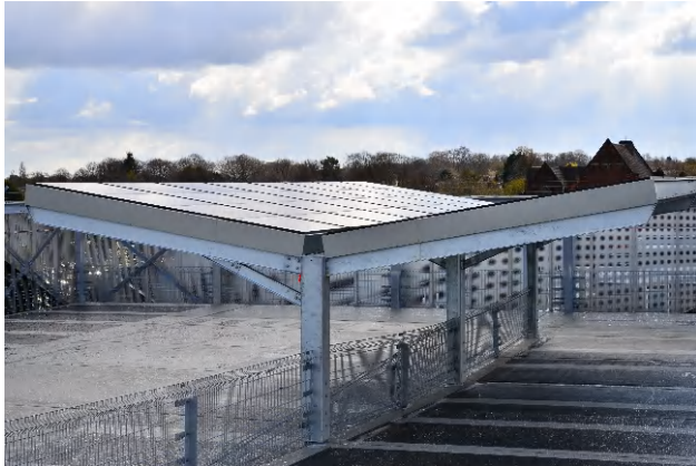
PV panels on the upper parking deck also provide shade
