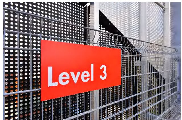
Open-weave facade provides natural ventilation
